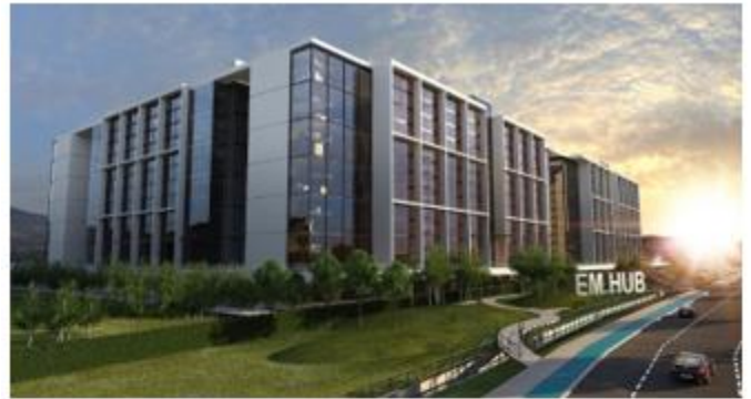
ActivePure is installed throughout Em Hub Kota Damansara
